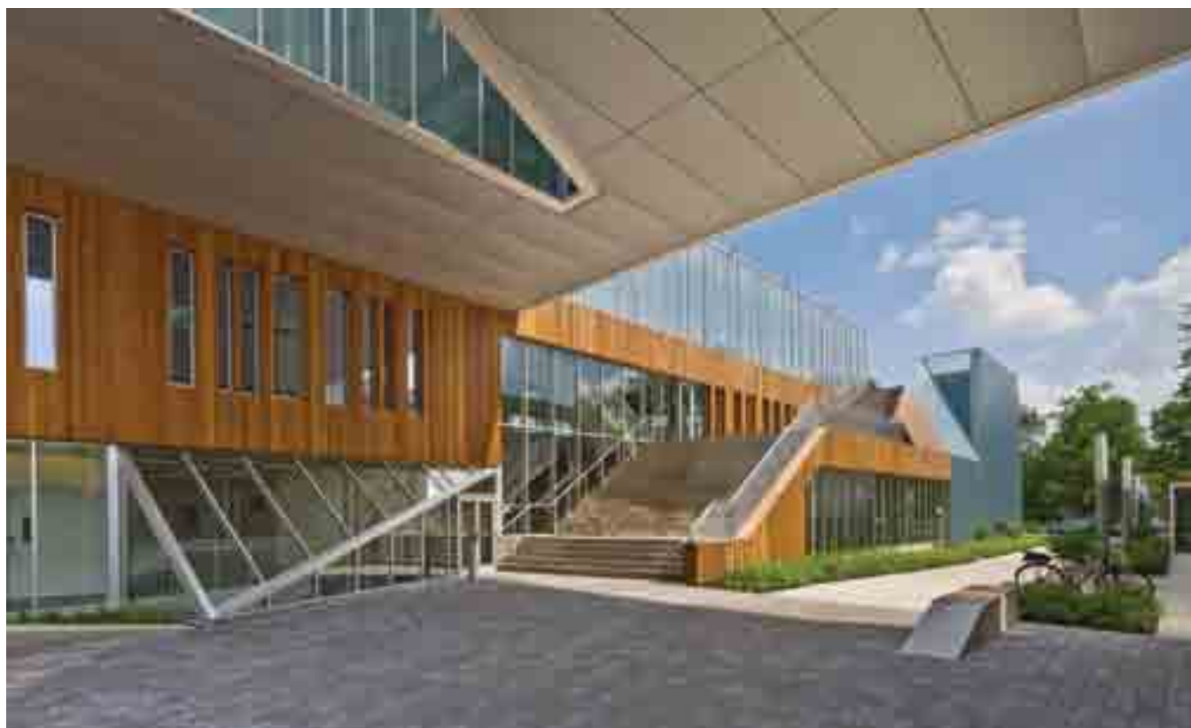
INSTRUMENTAL MIX Exterior materials include Brazilian ipé hardwood siding, a glazed curtain wall system and a custom stained-aluminum rain screen system.
