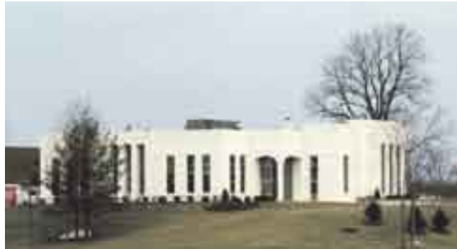
HOME BUILT Geis Companies, which employs 60 team members, is headquartered in Streetsboro.
